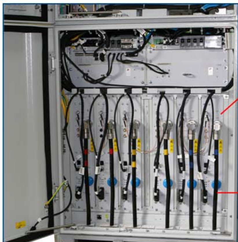
CPRI electrical cable on the RFU side
